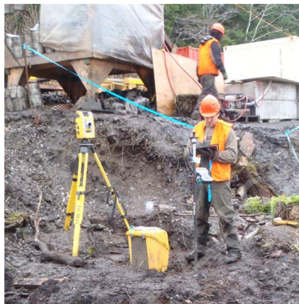
FIGURE 2: A CREW MEMBER RECORDS DATA USING A TABLET COMPUTER AND A ROBOTIC TOTAL STATION.
